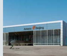
Ameco A380 Hangar Peking, China
